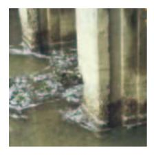
Figure 3. Corroded concrete due to sulphuric acid [nrm, 2002].
